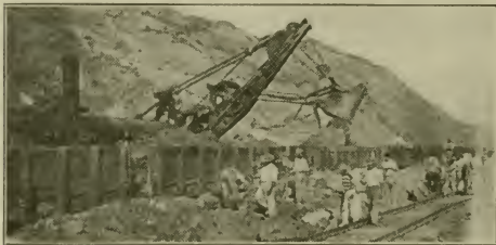
STEAM SHOVEL AT WORK IN CULEBRA CUT.
